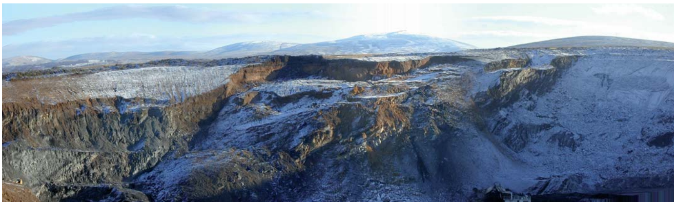
Massive failure of endwall of opencast coal site
