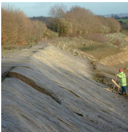
Progressive buttressing in progress
