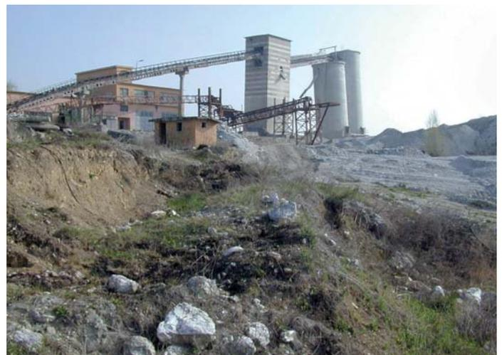
Large landslide causing silos to tilt
