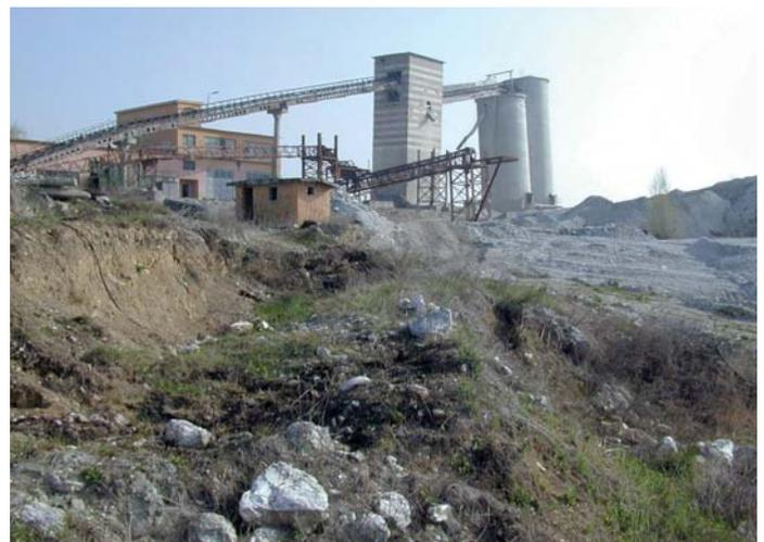
Large landslide causing silos to tilt
