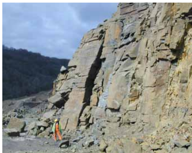
Geological and geotechnical mapping
