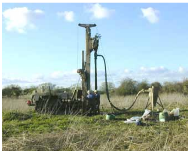
Site Investigation: Rotary drilling
